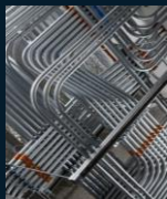
Conductors in Riser Conduits thru Building
