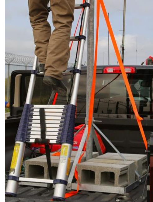
10x Tylon small ballast NPRMs (36"x36") shown knocked down on left along side rubber mats. One 36x36 NPRM assembled with 20cm concrete blocks on right.
