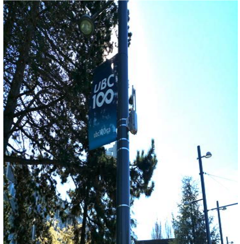
AP1572 shown mounted to 8" diameter pole – providing power and connection to CCTV
